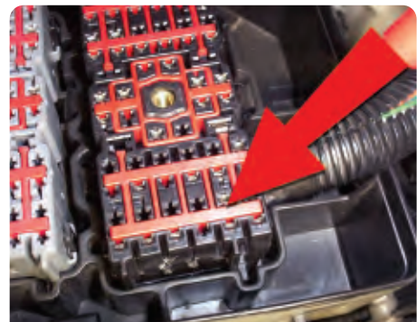
Damaged terminal in Connector 2 (viewed from top, with electrical center board removed)
