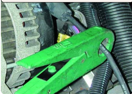
Correct current probe connection at generator
